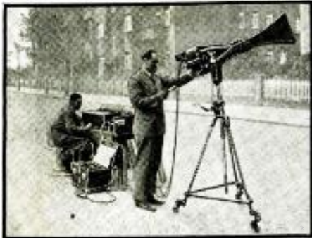
A new Telefunken transportable 20-W. P.A. system in operation. All the components of this device are contained in 2 ordinary-size trunks. Darn clever, these Germans!
